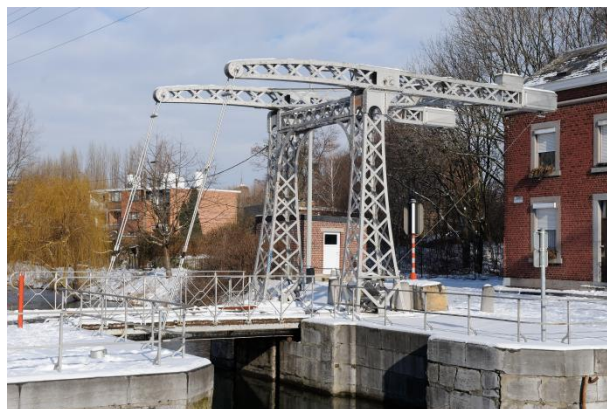
Pont-Levis des Aguesses (Photo G. Focant © SPW)
